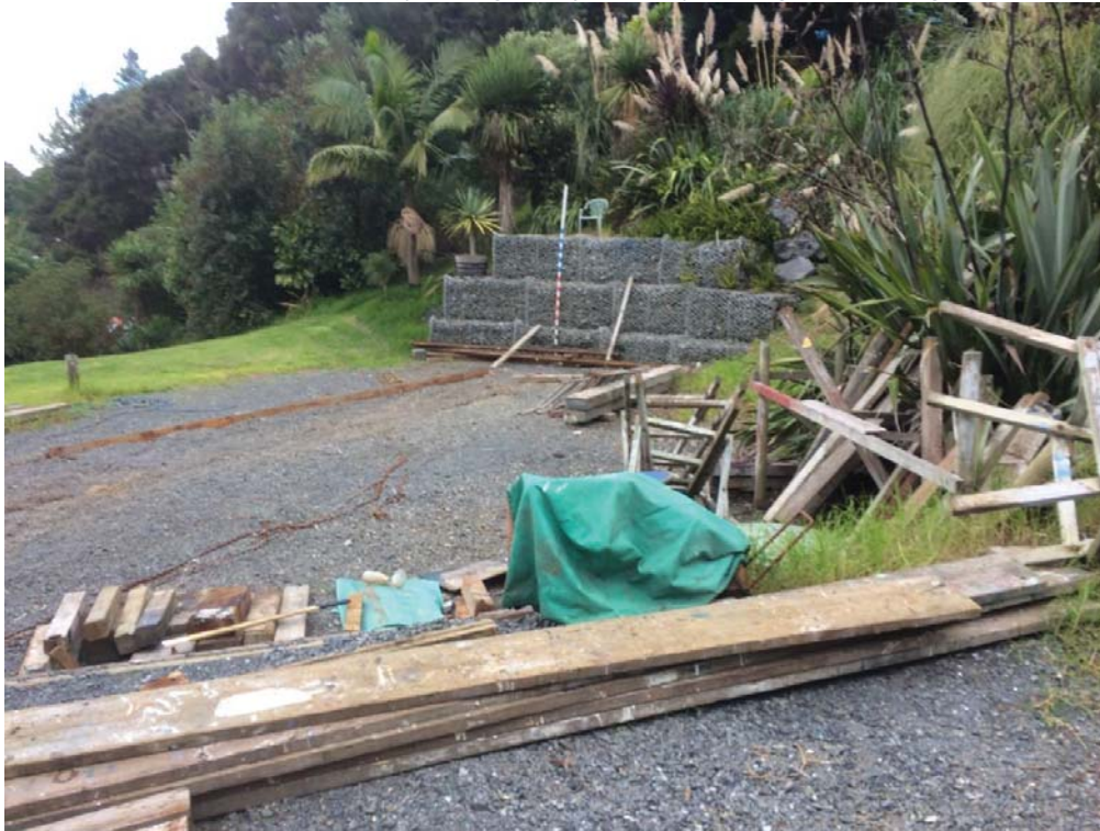
Figure 29 - Site Photo - Southern site boundary showing area of metallised yard and gabion retaining wall.
