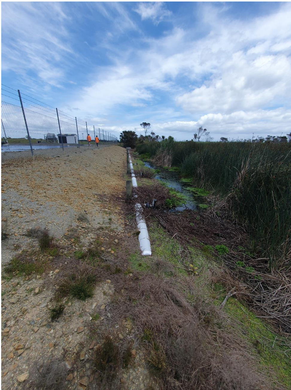
Figure 1 Whatuwhiwhi WWTP outlet diffuser, with nutrient tolerate wetland vegetation.
