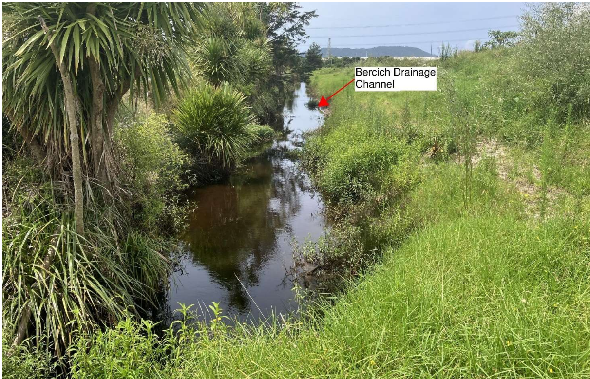
Figure 4-2: Bercich Drain running through the centre of Site 1.
