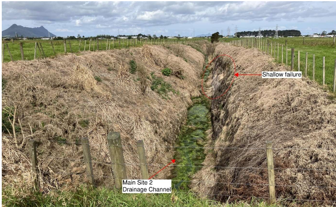
Figure 4-5: Main 4m deep drainage channel running through Site 2
