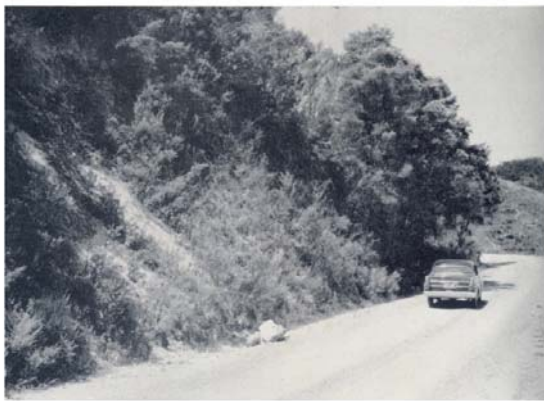
Material dislodged from an existing roadside slip at Kaingapiwai, on the Pupuke Road.
