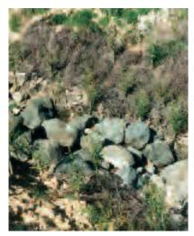
Rocks and willows below a flume to protect soil from the force of the water.
