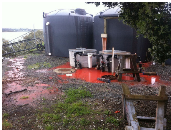
Plate 10. Unauthorised discharges from a boat maintenance facility, because of system failures, maintenance issues or leaks can cause metal contamination.
