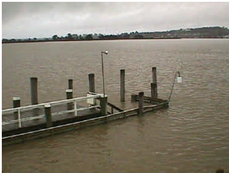
Tidal monitoring station at Dargaville
