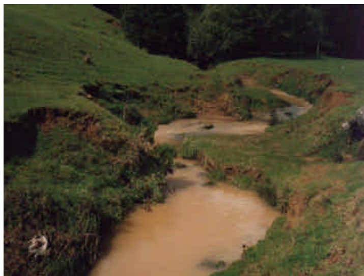
Typical Northland stream passing through farmland suffering from bank erosion
