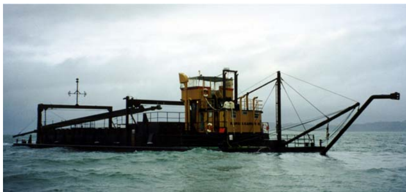
Dredge operating on the Kaipara Harbour
