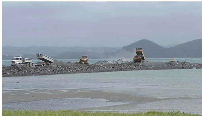
Reclamations underway for the new deepwater port at Marsden Point
