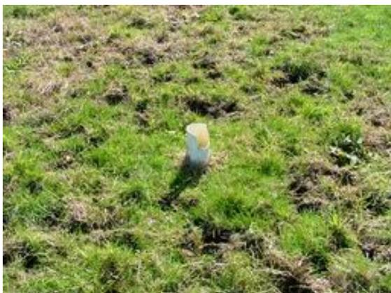
Photo: badly constructed bore
