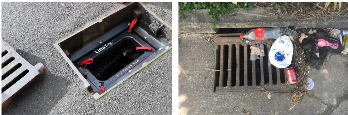
Figure 10. Example of a LittaTrap (proprietary device) installed within an existing roadside stormwater drain. These provide an additional filter that traps smaller pieces of litter that would otherwise flow through the grate.
