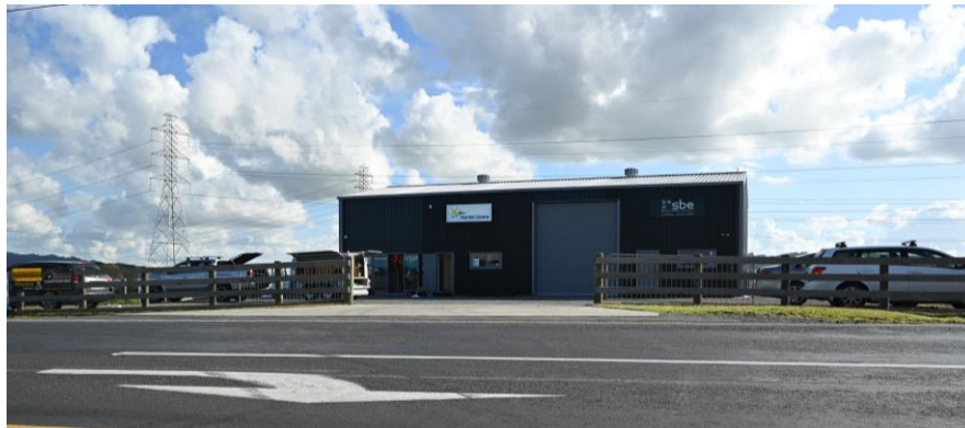
Photograph 5: The recently constructed small industrial building that sits amidst the eastern margin of the Site. This lies on an allotment that has just been subdivided from the title. Note high tension pylon corridor situated in the midst of the southern part of the Site in the background.
