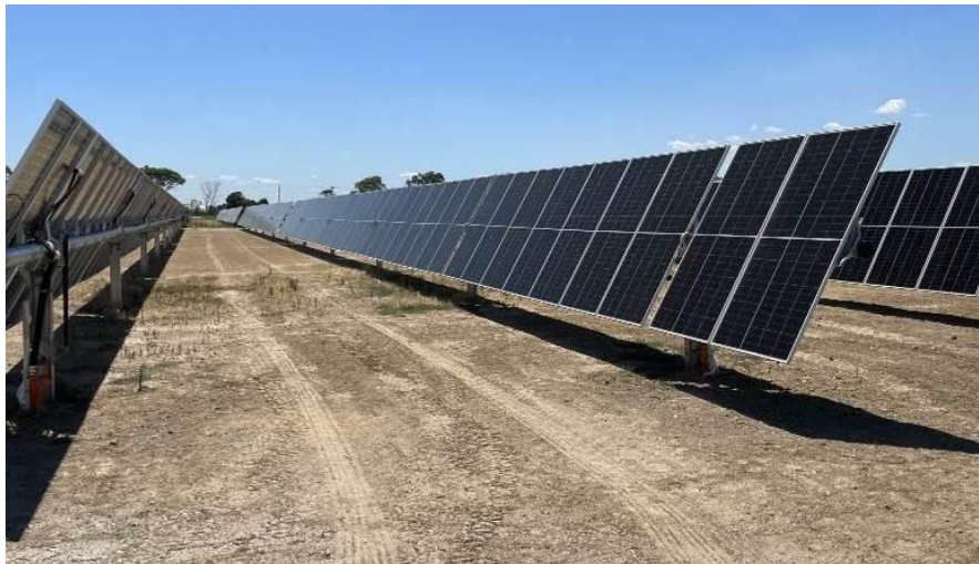
Photograph 11: A typical fixed axis solar array installation. The panels proposed by the application would be mounted higher than this example, particularly in areas that are prone to inundation. Image source: Meridian
