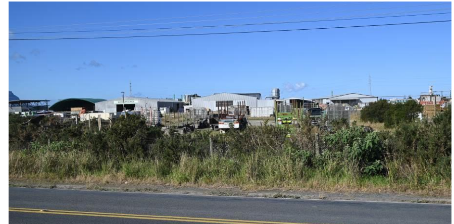
Photograph 6: Light Industrial zoned development near Lakeside Park Road, as seen from Marsden Point Road.
