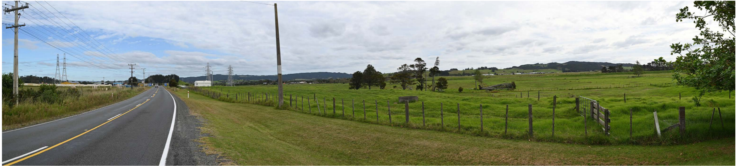
PANORAMIC PHOTOGRAPH OF CURRENT SITUATION VP08 | MARSDEN POINT ROAD
