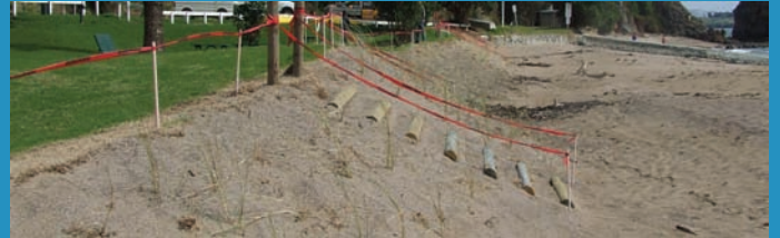
After... the beach following dune restoration.
