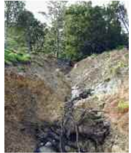
Actively eroding gully.
