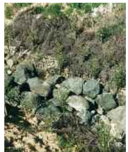
Rocks and willows below a flume to protect soil from the force of the water.
