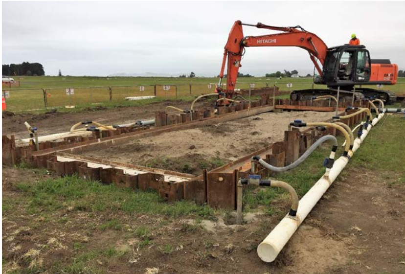
Photo 1: A sheet piled and well pointed site ready for excavation.
