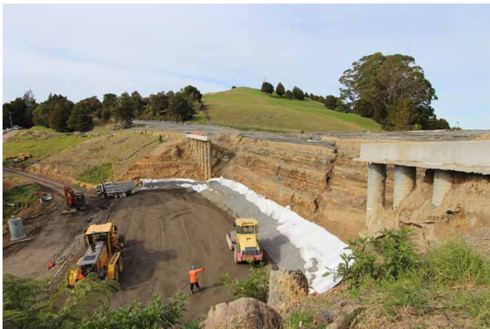
An expensive problem to fix – slip repair on SH1 near Maromākū, following July 2014 storms (Source: NZ Transport Authority).
