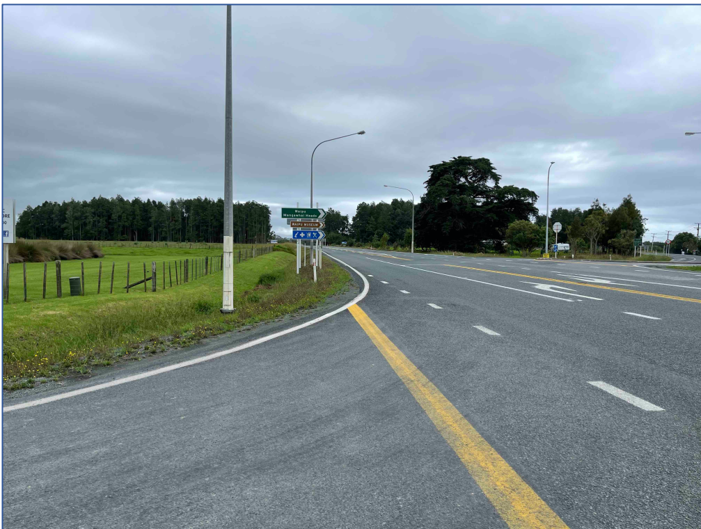
Figure 6: SH1 looking to the north from Millbrook Road
