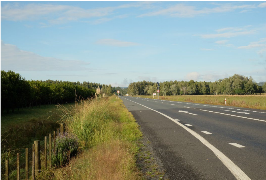
Figure 4: East side of SH1 close to the intersection of Shoemaker Road with SH1; approximately 1000m north of the north-east corner of the stie (photo RKL - 19 03 2022)
